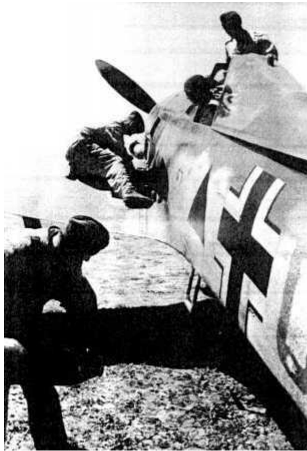
Figure 5 - SchG.1 - 2 Staffels' Red "C" receives last minute adjustments to the inboard gun by "Blackman" (mechanics), whilst another brings out a bomb for C/L rack.
