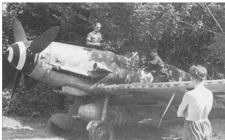
Figure 5 - A I Gruppe Me 109G-10 with drop tank for extended range, late 1944, note absence of "Udet" badge.
